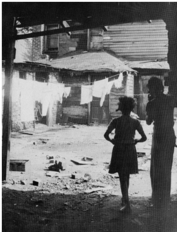
Figure 3. North side of Indianapolis slum conditions. Image Credit: Indiana Historical Society
