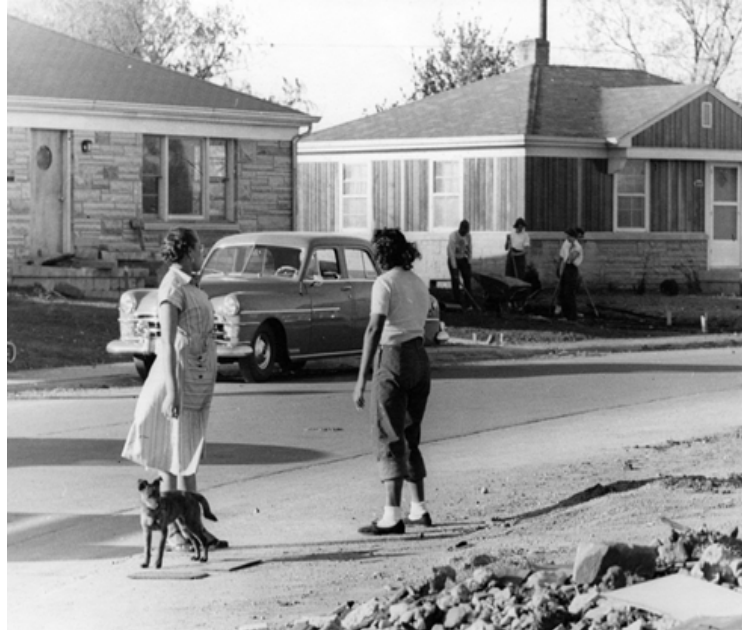
Figure 13. Construction of the Fall Creek Self-Help Homes. Image credit: Indiana Historical Society
