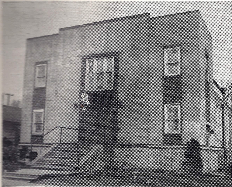
Twenty Second Street and Columbia Avenue Indianapolis, Indiana
